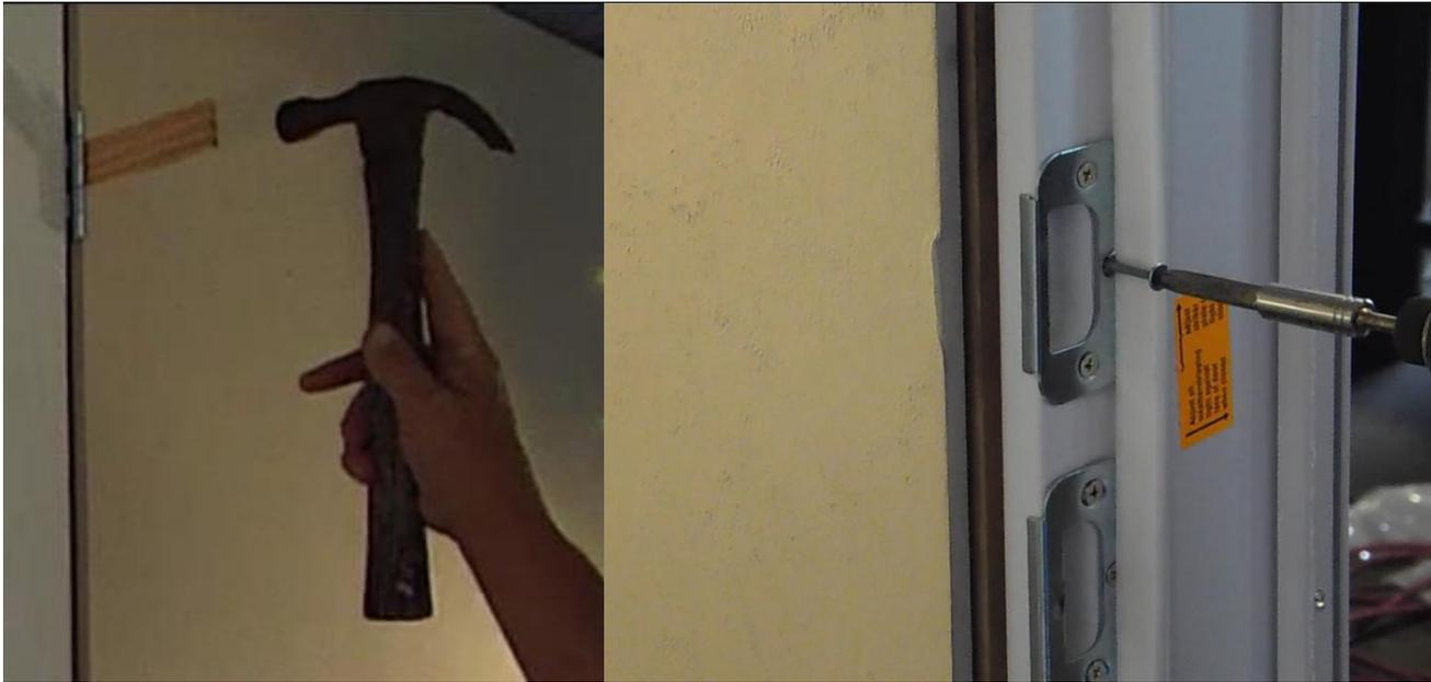
8. If the gap between the jamb and stud is greater than  $\frac{1}{4}$ " and if the jamb is bowed out at the lock, it will be necessary to shim behind the jamb.
