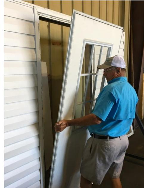
3. Do **NOT** open the door or remove shipping clips or shims before installation. Opening the door before installation will destroy the proper squaring of the door. If shims are not in place, position one shim at the bottom of the door core butting the striker side frame and underneath the core. Position the other shim near the striker plate between the core and the frame.
