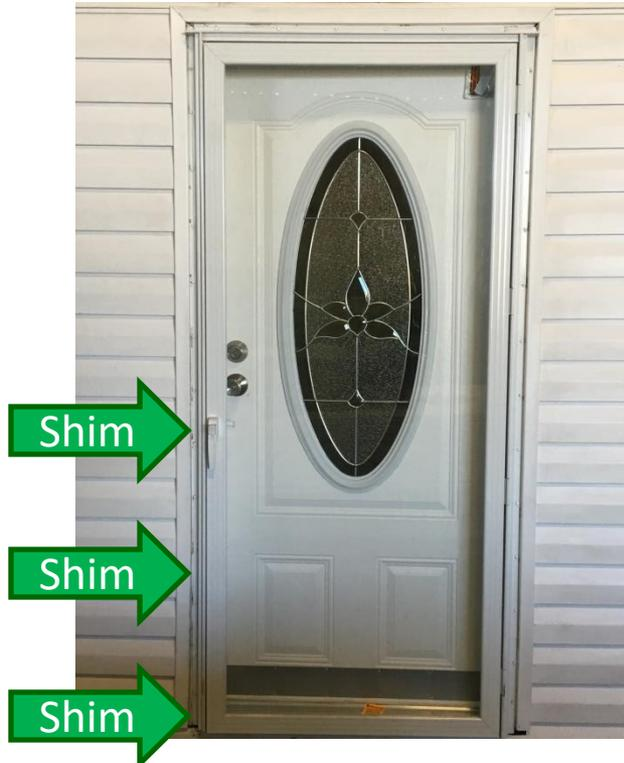
3. Do **NOT** open the door or remove shipping clips or shims before installation. Opening the door before installation will destroy the proper squaring of the door. If shims are not in place for the storm door, position one shim in the striker location and another 2/3 the way down. Position a third shim on the inside core under the sweep and butting against the lock side jamb.
