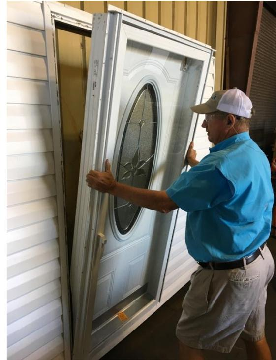
4. Grasp the frame on the sides, lift and tilt towards you. Insert the door assembly carefully into the rough opening. Making certain the door sill is secure on the floor.
