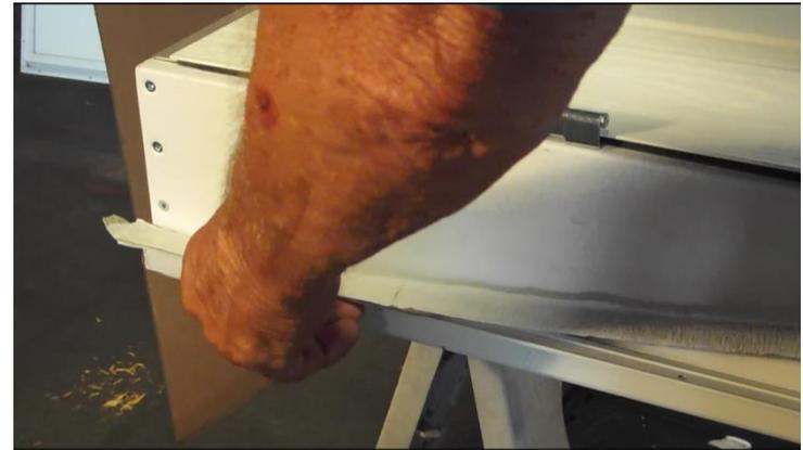
1. Making certain all mounting surfaces (siding seams included) are securely fastened and flat around the perimeter of the rough opening. There should be no obstruction in the opening (i.e. nails, staples, nailing strips, belt rails, etc.).
